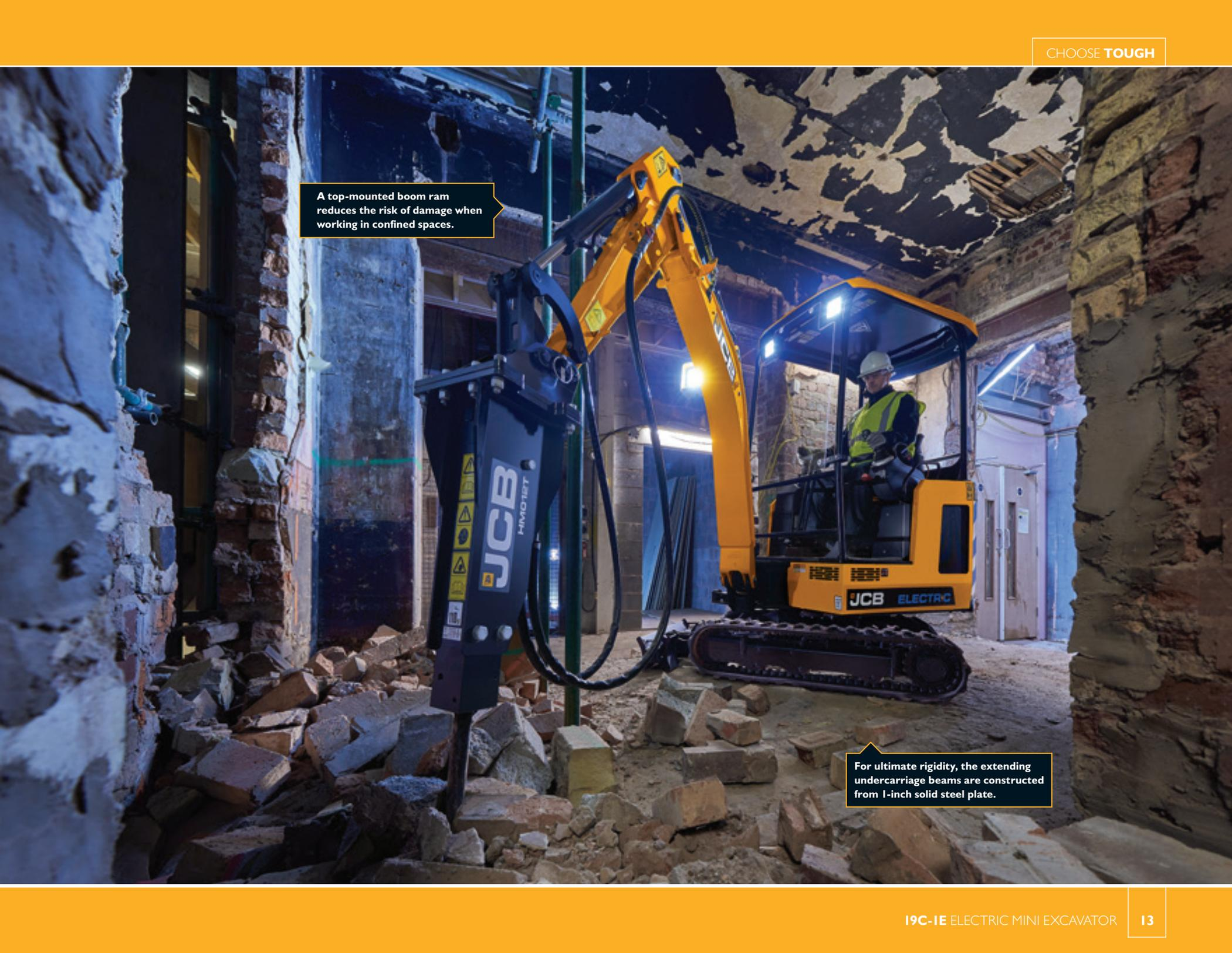
A top-mounted boom ram reduces the risk of damage when working in confined spaces.
